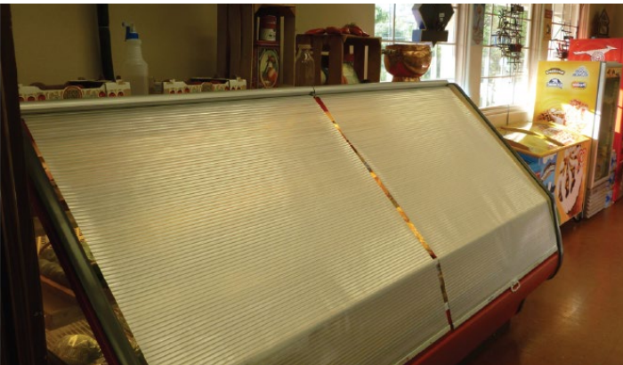
Night covers for reach-in refrigerated display cases are shown at Frontier Mart, Corrales, NM.
