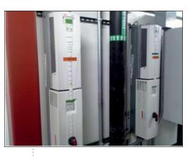
Institutions can often **reduce their** electricity use and costs by 5 to 15 percent or more by improving the efficiency of their motor-driven systems, according to the US Department of Energy. The variable speed drives (VSDs) shown here are installed at the University of New Mexico.
